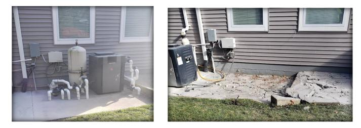
• Call in for inspection, if needed. Some Municipalities require this to ensure nothing is buried illegally. For abandonment in place, just about all municipalities will allow only the broken concrete (or brick) to be left in the cavity provided its broken down to basketball sized or smaller pieces.
