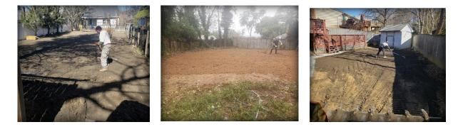
• Lightly rake in the seed to lightly cultivate the seed into the soils. Cover entire area with straw. Repair access point to work area, removal of silt fence, if installed and then call in for the final inspection
