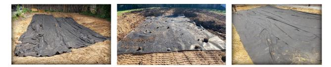
• Add common fill dirt up and compact frequently in lifts up to 12", repeatedly.
